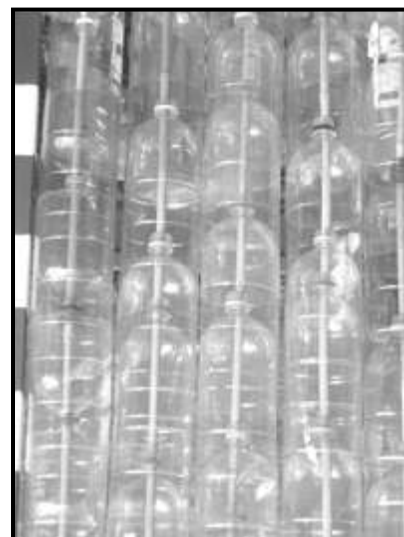
Close up showing the plastic bottles threaded on bamboo canes
