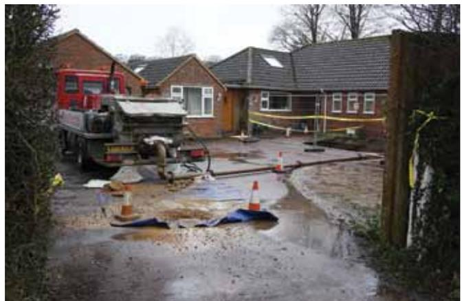
So what caused the sinkhole (or the Lupole as it quickly became christened)? The theory is that 50 years of the gutter soakaways eroded the sandy soil under the clay, creating a cavity that chose that moment to collapse, probably because of all the recent rain. Where it all went, they are not sure although the old chalk mines may have played a part. But hopefully
